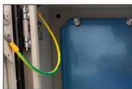
Grounding screw More aesthetically pleasing and safer
