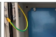
Grounding screw More aesthetically pleasing and safer
